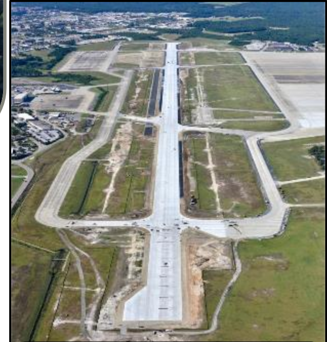
Pope Army Airfield Runway Replacement Ft. Bragg
